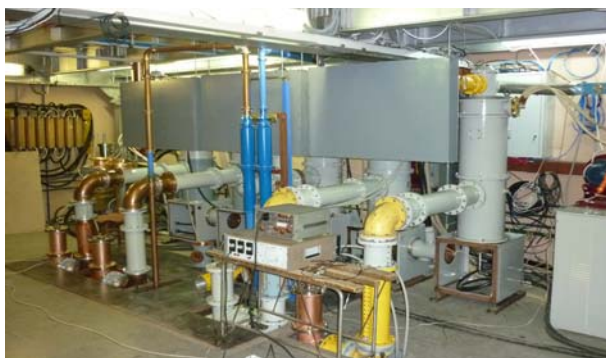
Fig.5 RF generator of the ILU-14 machine in the BINP.
